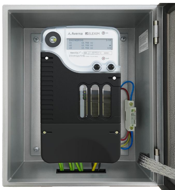
Figure 11 Real installation of device MeVOLT®
